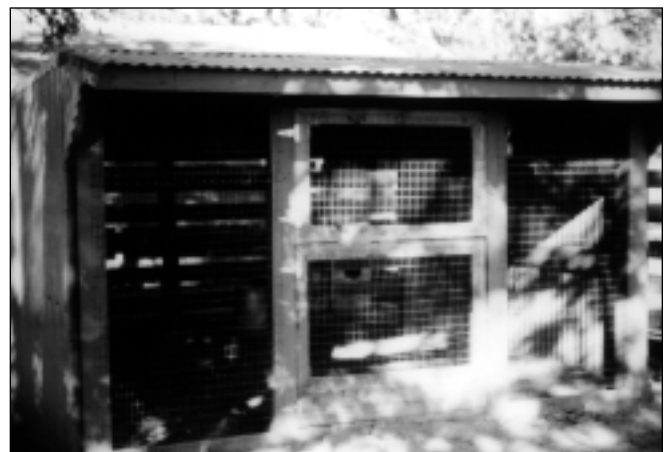
A typical building used for growing broilers or roasters for a youth project.
